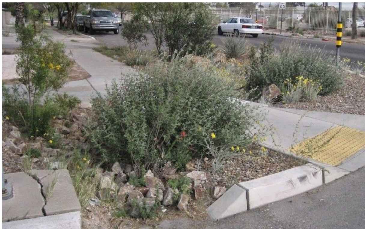
A type of green stormwater infrastructure practice integrated into a curb bump-out: runoff from the street is diverted into the planted area opposed to entering the storm drain. Source: U.S. EPA Flickr account
